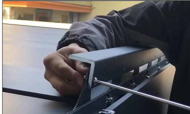
2. Preinstall the connecting rod with the hex wrench
